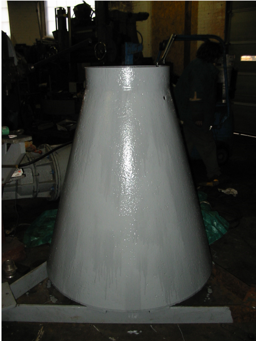
Fresh paint applied to newly patched inner cone.
